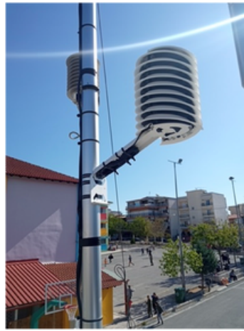
KORDELIO (WEST SIDE)
